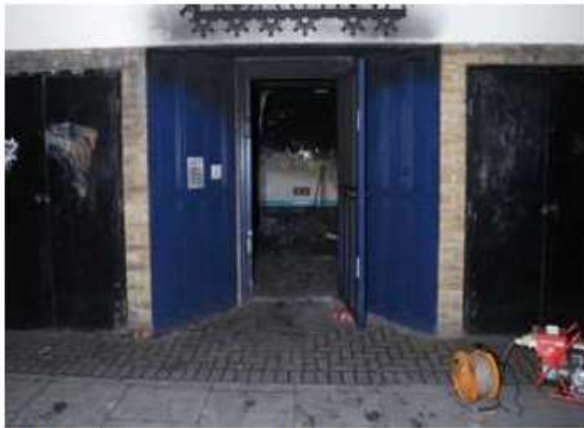
View of front communal entrance
